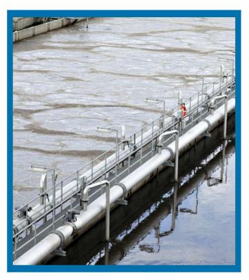
The Zuluf project consists of a water treatment plant with a 185,000 m³/day capacity supporting water injection for the Zuluf Onshore Oil Facilities project, located in the Arabian Gulf, 240 km north of Dhahran.
