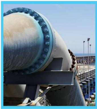
The Centinela water transportation system project, a strategic initiative, involves the acquisition and operation of a 144 km long water pipeline that transports 1,194 lps (110,678 m3/day), supplying seawater approximately 60 km north from the mining site at Michilla, where Centinela's port is located. The project also includes the construction and operation of a new pipeline 144 km long and 650 lps (56,333 m3/day) parallel to the existing pipeline to provide seawater.
