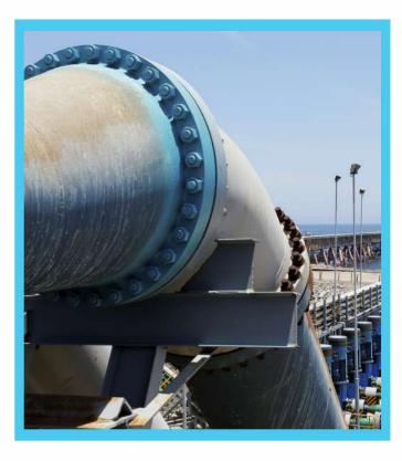
The Centinela water transportation system project, a strategic initiative, involves the acquisition and operation of a 144 km long water pipeline that transports 1,194 lps (110,678 m3/day), supplying seawater approximately 60 km north from the mining site at Michilla, where Centinela's port is located. The project also includes the construction and operation of a new pipeline 144 km long and 650 lps (56,333 m3/day) parallel to the existing pipeline to provide seawater.
