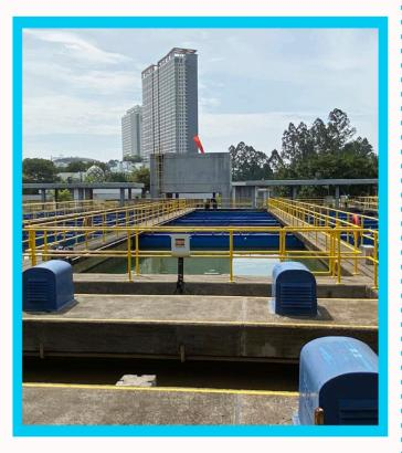
Tirta Kencana Cahaya Mandiri is a water company that operates a drinking water treatment plant under RUOMT (Rehabilitation, Uprating, Operation, Maintenance, and Transfer) with a total capacity of 140,000 m³/day under a 20-year concession contract.
