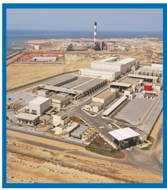
The Shuqaiq 3 desalination plant, located on the coast of the Red Sea in Saudi Arabia, is one of the world's largest reverse osmosis desalination plants. With a nominal production capacity of 450,000 m³/day, equivalent to 180 Olympic-size swimming pools, the plant supplies both the population and the agricultural and industrial activities of the provinces of Asir and Jizan, which are home to nearly 4 million people.
