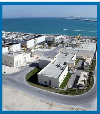
The Muharraq project is a 100,000 m<sup>3</sup>/d state-of-the-art wastewater treatment plant with a sewer conveyance system in the Muharraq catchment area. The conveyance system includes the first 16.5 km deep gravity sewer trunk pipeline in the GCC region and a wastewater collection network.
