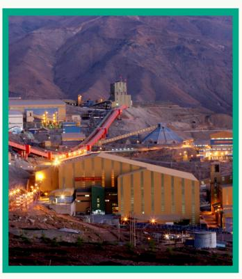
Almar Water Services Latam performs the operation and maintenance of the water treatment plant that is drained from inside the tunnel of the Codelco El Teniente Division, which allows the recovery of about 12,000 cubic meters of water per month to process copper ore.
