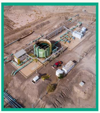
Since 2018, Almar Water Services Latam has been developing activities associated with operating and maintaining a water impulsion and catchment system consisting of five deep wells, four intermediate pumping stations, and 68 km of line. With an average pumping capacity of 90 l/s, this system allows our client to provide operational continuity and focus its active efforts on its core business.
