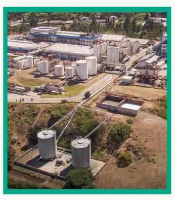
One of the most important clients in the chemical industry is BASF, located at the Concón site. Our service operates and maintains the wastewater treatment plant using a physical-chemical system plus a biological treatment system that allows the client to discharge the treated water in compliance with the quality requirements of Supreme Decree 90.
