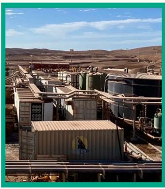
Antucoya Mining's desalination plant has been operating since 2011, producing 2,930 cubic meters of water per day for the industrial client Antofagasta Minerals, located in northern Chile. Using reverse osmosis technology, the plant captures seawater, which is subsequently treated in different phases, producing quality process water in sufficient quantities.
